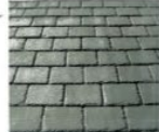
Natural slates to plot 4 main dwelling roof area and roof areas of cart-lodges serving plots 1 and 2.
