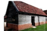
Red brickwork plinth with black timber weatherboarding over.
