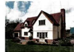
Red brickwork plinth with painted render over.
